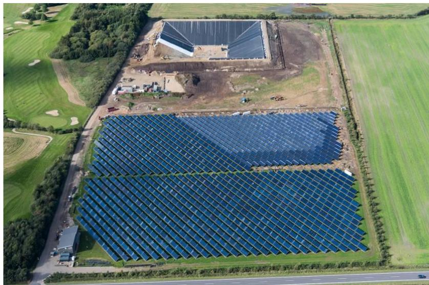
**Figure 16 - Toftlund District Heating. 27,000 m<sup>2</sup> solar panels and 70,000 m<sup>3</sup> water. The facility will cover approximately 45 % of the total heating needs of the 1,033 individual customers.**
