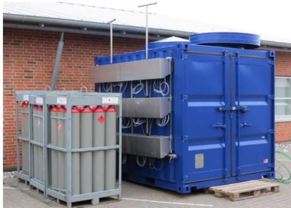
**Figure 15 - A 50 kW LT-PEMFC CHP hydrogen unit from Dantherm Power.**
